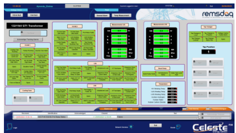
Substation Transformer Mimic
